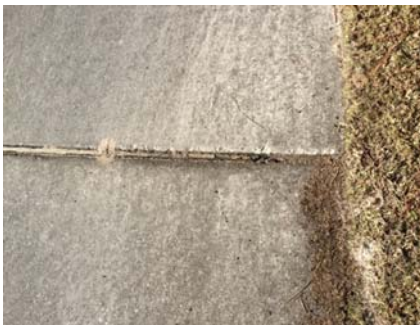
Chula Vista cart path repairs
