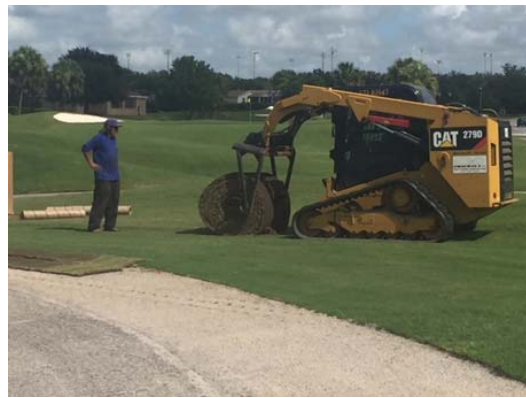
Hawkes Bay greens & tee renovations
