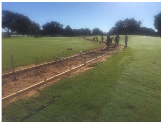
Silver Lake cart path renovations
