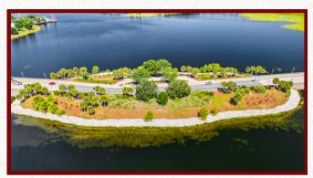
work was to protect the island shoreline by strategically installing riprap, a key defense against water's erosive forces, as well as rock underlayment to provide maximum protection against storm surge and erosion.
